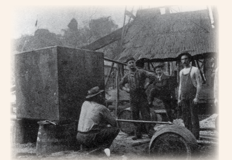
400 gallon oil storage tank at Guapo, claimed to be the earliest oil storage tank built in Trinidad
