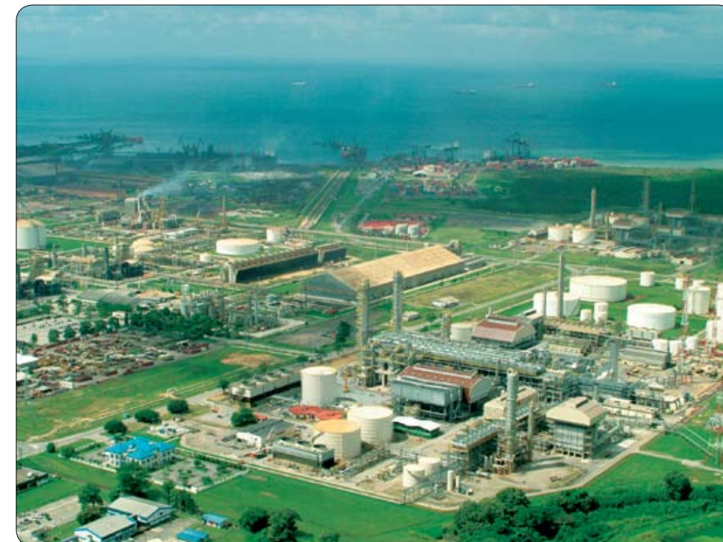
Point Lisas Industrial Estate: experiencing a new wave of downstream gas development
