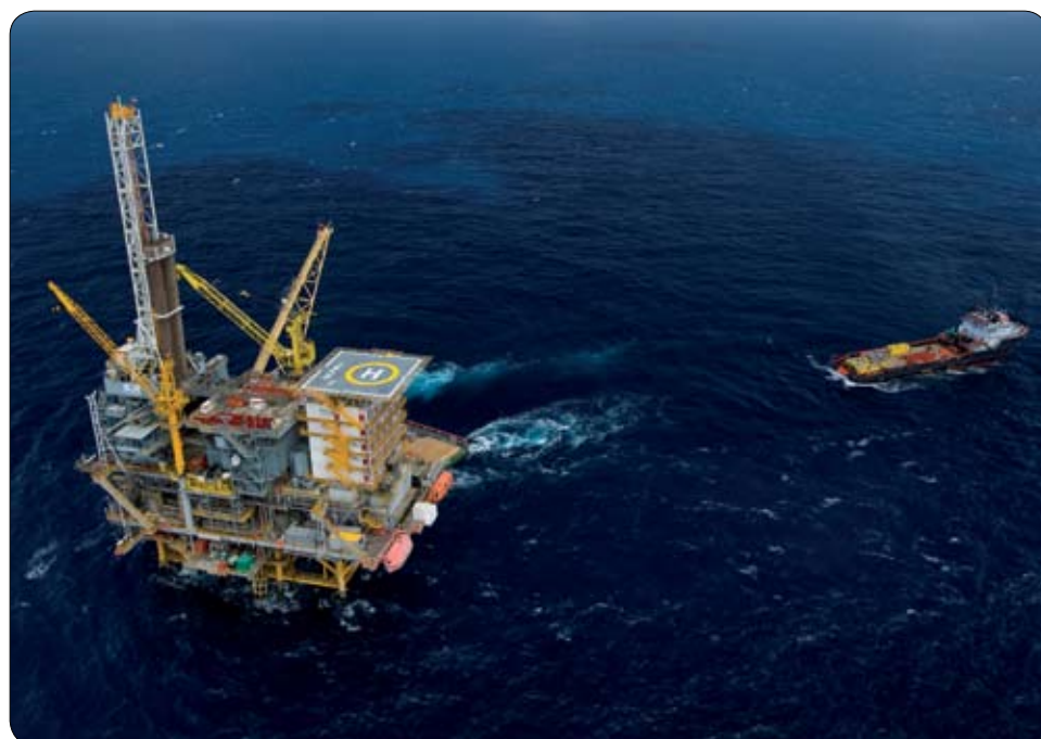
BG's Hibiscus platform: the company's Manatee well in block 6d confirmed the existence of cross-border gas reserves between Trinidad and Tobago and Venezuela
