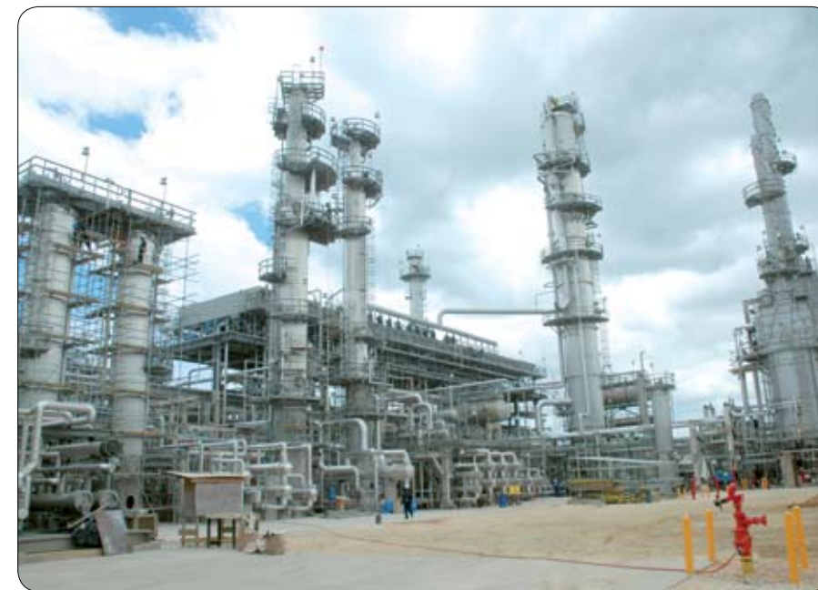
Petrotrin's Pointe-a-Pierre refinery is undergoing a US$850 million upgrade
