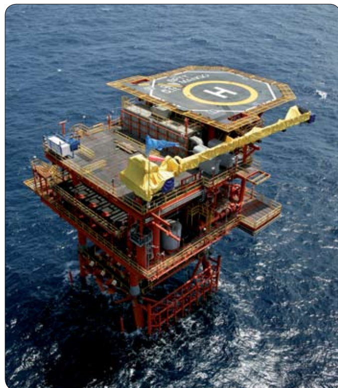
bpTT's Mango platform off the east coast of Trinidad
