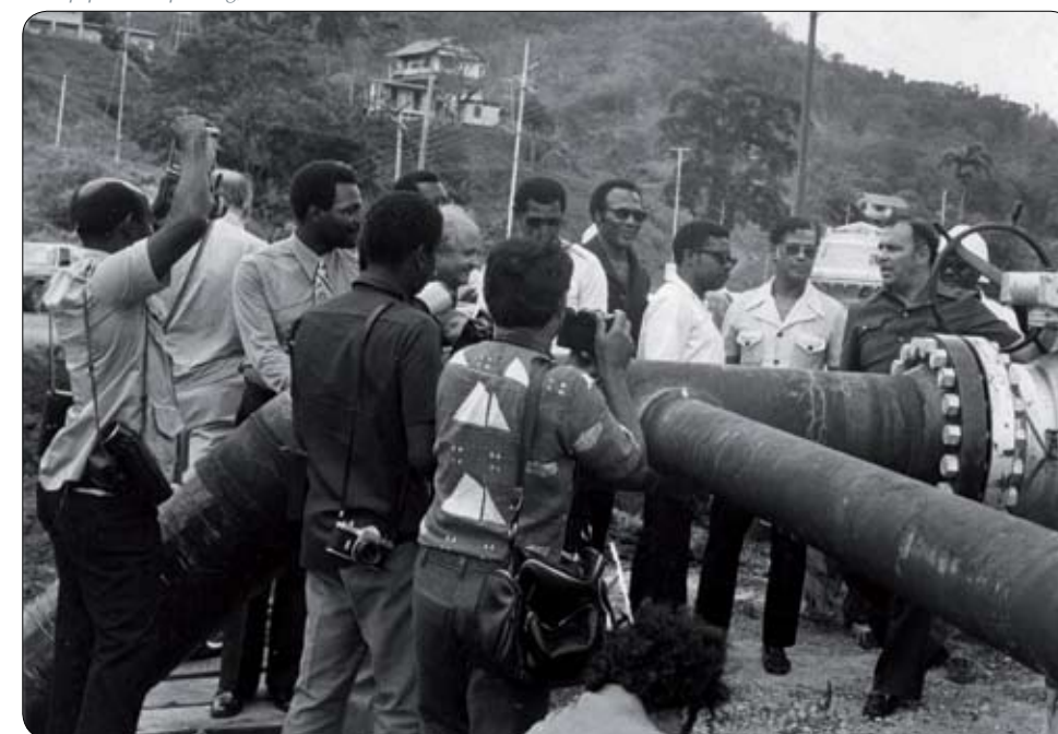
Gas pipeline opening, 1964
