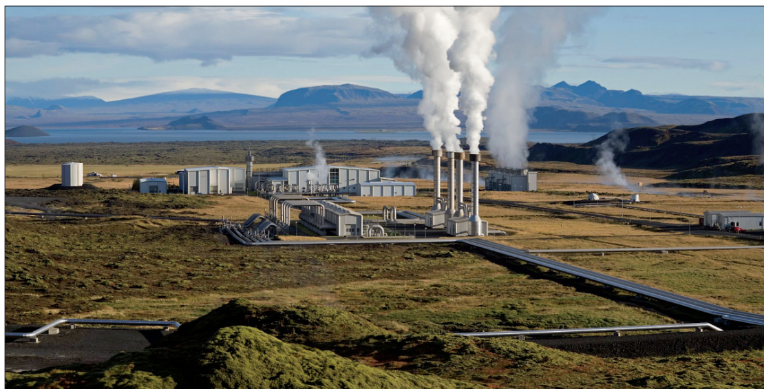
Nesjavellir Geothermal Power Station in Iceland: the station produces approximately 120MW of electrical power and delivers around 1,800 litres of hot water per second, servicing the hot water needs of the Greater Reykjavik Area
