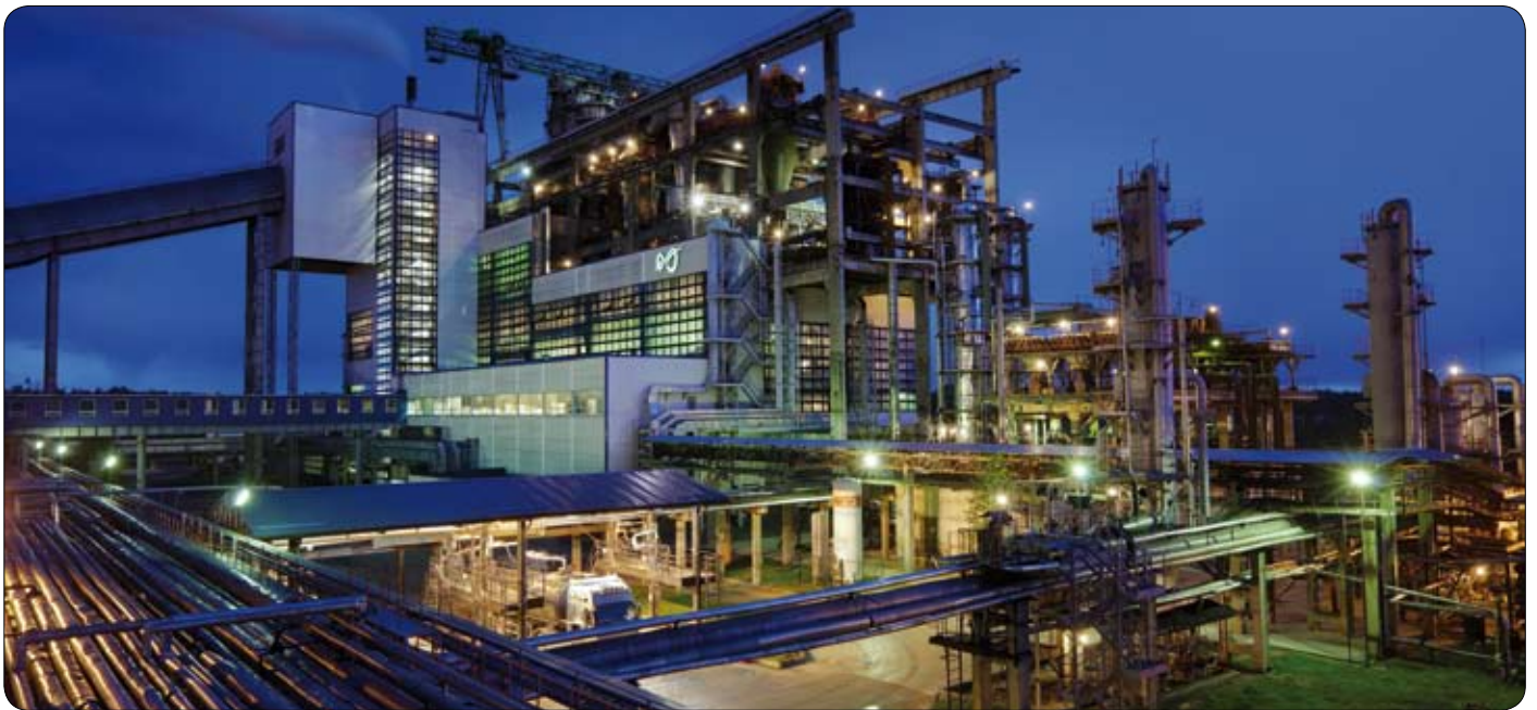
Eesti Energia Oil and Gas's Enefit 140 Plant in Narva, Estonia. The plant currently operates two production lines, each consuming 140 tonnes of oil shale per hour. The new Enefit 280 plant (consuming 280 tonnes per hour) is currently under construction
