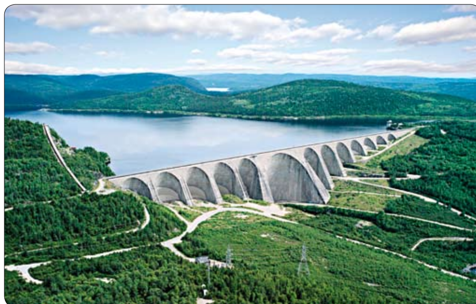
Manic-5, a 1,596MW generating station on the Manicouagan River, was commissioned in 1970-71
