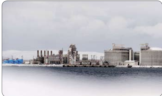
Snøhvit is Europe's first export facility for liquefied natural gas (LNG) and the largest-ever industrial project in northern Norway. Natural gas produced from the Snøhvit, Albatross and Askeladd fields in the Barents Sea are received and processed at the plant (pictured) on Melkøya island outside Hammerfest
