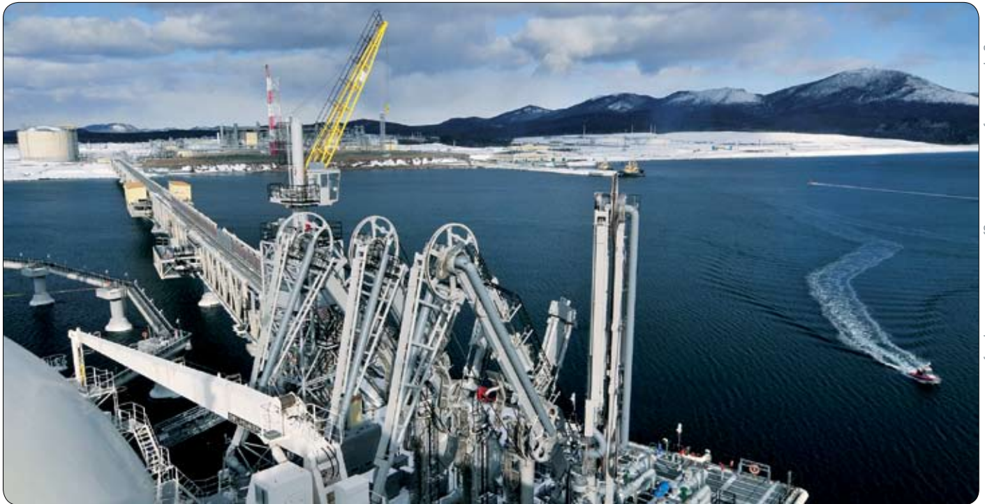
Figure 1: Russia's Sakhalin II project is the country's first LNG production plant, consisting of two trains capable of producing 9.6mta of LNG
