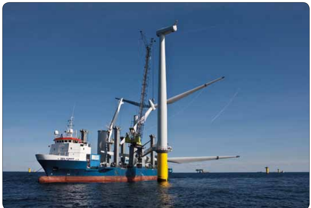
Assembly of a turbine in the Horns Rev wind farm in the North Sea
