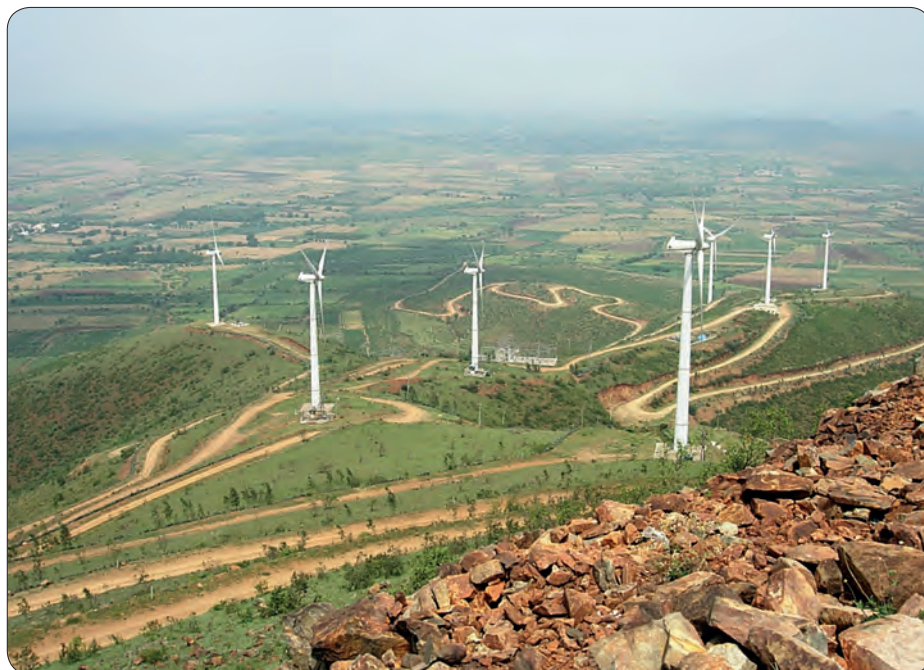
India's wind sector is the world's 5th largest with over 16 GW of installed capacity
