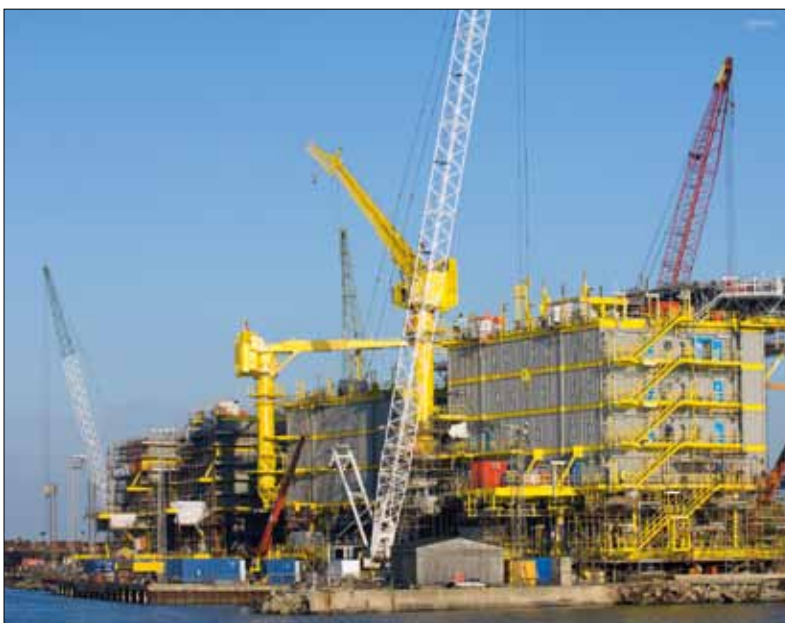
CONSTRUCTION AS WELL AS EXTRACTION CONTINUES IN THE NORTH SEA
