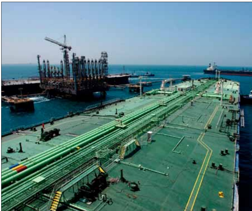
A supertanker berths at the Ras Tanura Sea Island Terminal, the main Saudi loading port
