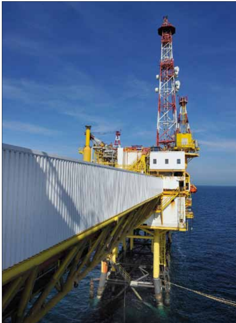
Production and gas processing platform in the North Sea off the Netherlands
