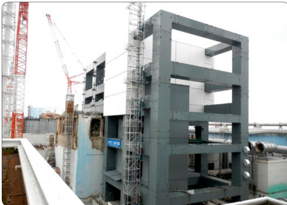
Steel frame for fuel removal at Unit 4 of Fukushima Daiichi Nuclear Power Station
