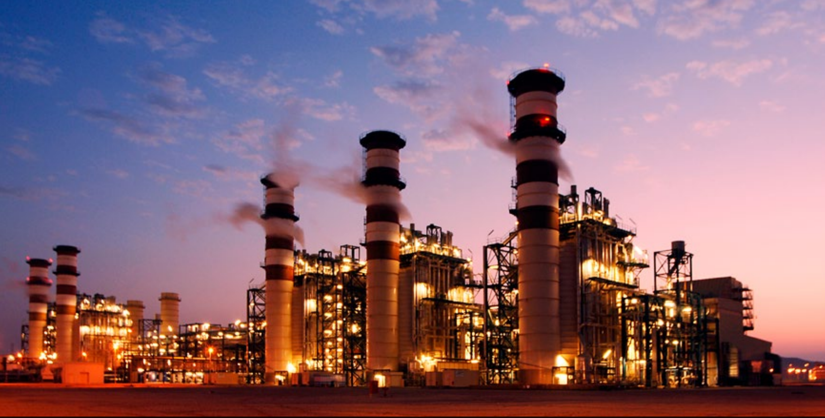
Oil refinery, Bahrain: The Kingdom was the first GCC nation to discover oil, in 1931
