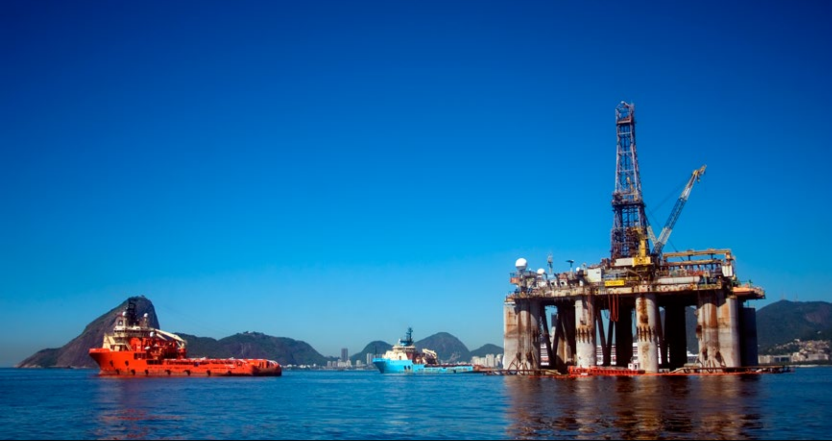
Petrobras platform, Guanabara Bay, Rio de Janeiro, Brazil
