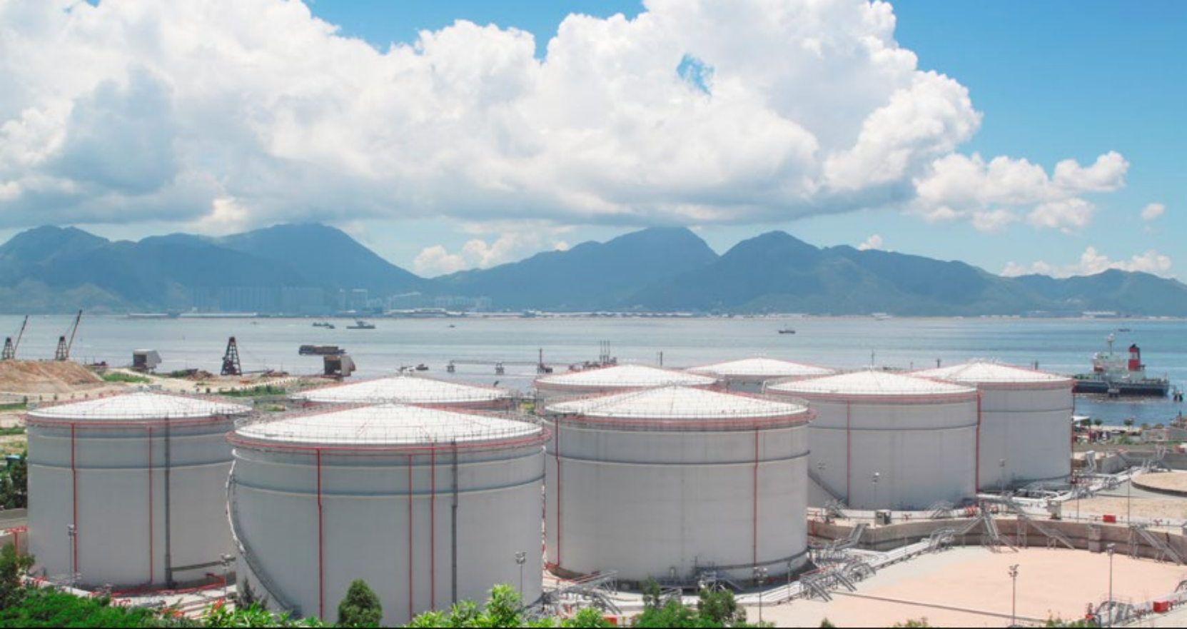
Gas storage tanks, Hong Kong Special Administrative Region, China
