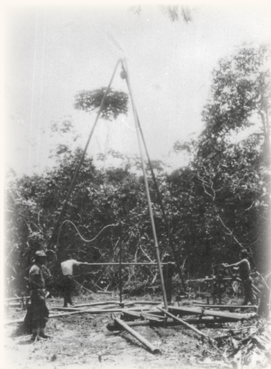
Drilling by muscle power at Tabaquite, 1928
