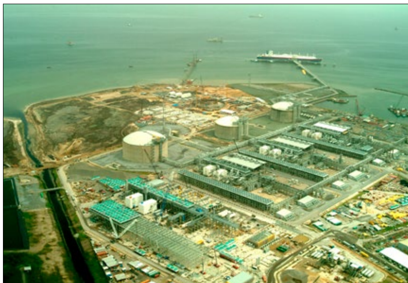
Aerial view of Atlantic LNG's Point Fortin site during the construction of Train 4
