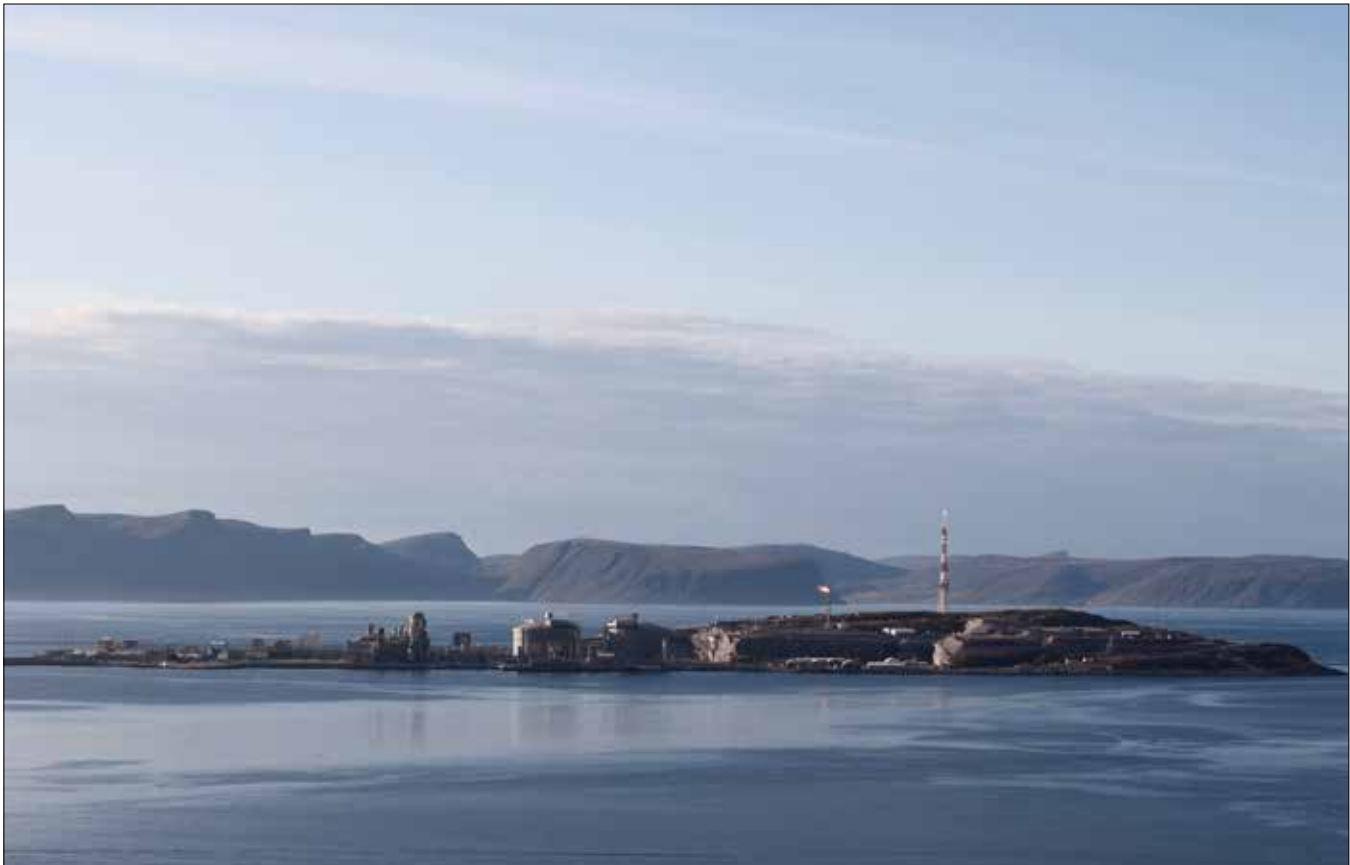
Energy processing island near Hammerfest, Norway
