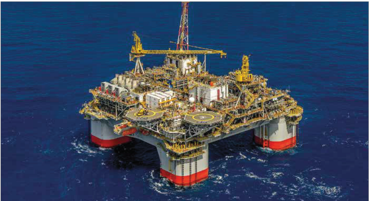
Chevron's Jack/St Malo floating production unit in the Gulf of Mexico, fed by the two oilfields of these names
