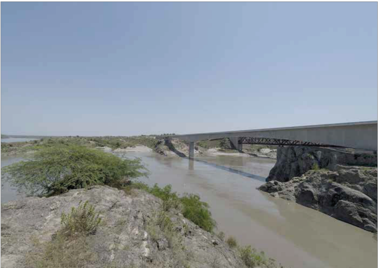
The Khushal Garh Bridge over the Indus River, built in Pakistan in 2016, with financial support from MOL
