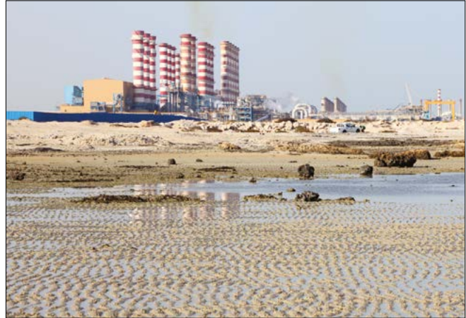
Natural Gas Power Station on the Coast in Qatar
