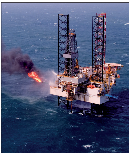
The Wil Superior drilling rig testing the Hai Su Den exploration well
