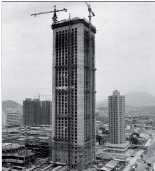
Shenzhen Special Economic Zone under construction in the early 1980s
