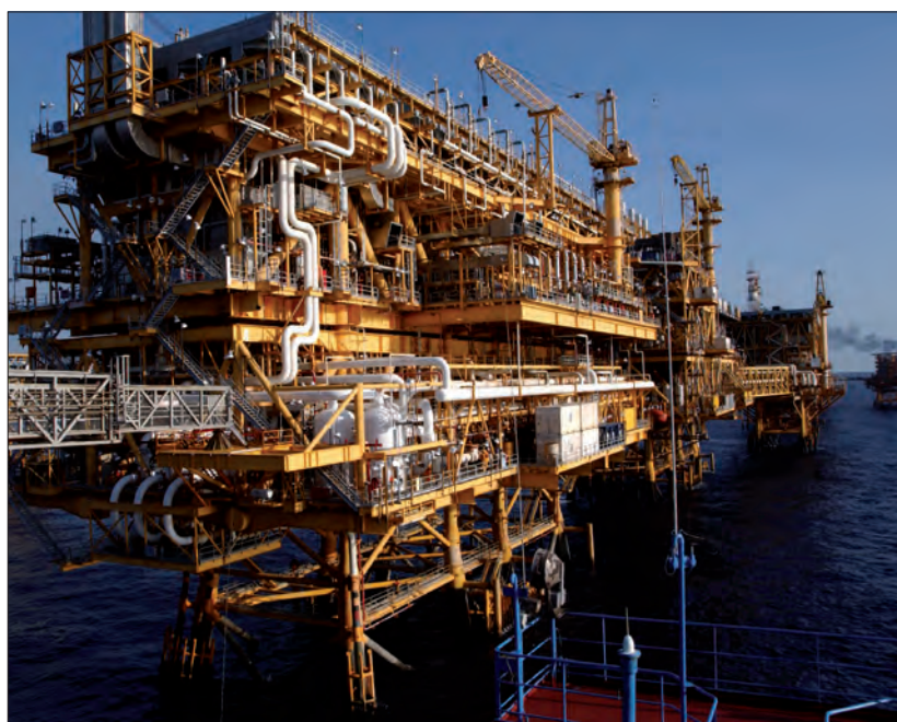
PEMEX offshore platform, Sonda de Campeche, Gulf of Mexico
