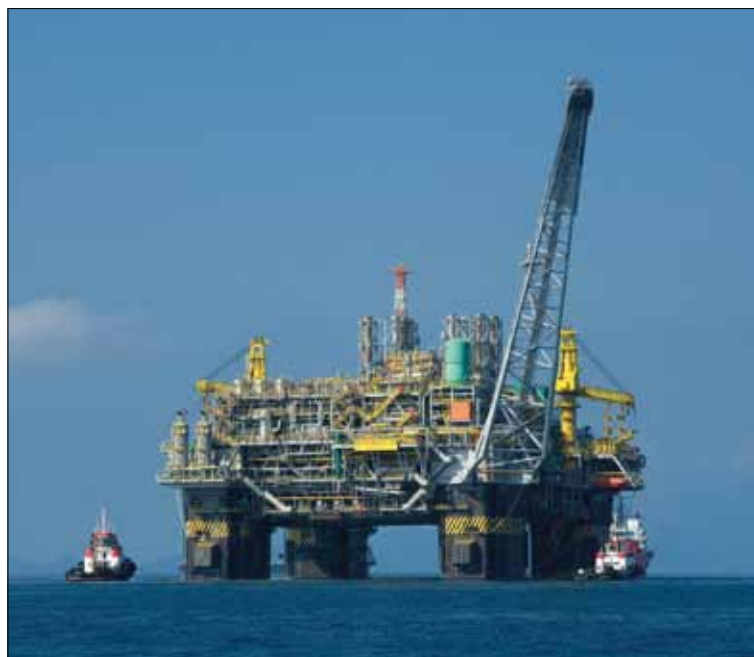
Petrobras's P-51 semi-submersible oil platform, which started production in 2009, is the first 100 per cent Brazilian-built platform
