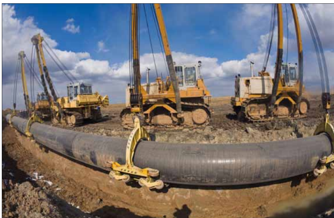
Oil pipeline under construction in the Mangistau region of Kazakhstan
