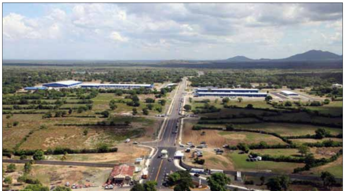
The Caracol industrial park has the potential to transform the economy of northern Haiti
