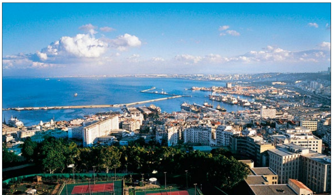
The bay of Algiers: North Africa's most important seaport
