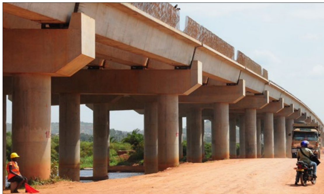
Construction of the Kampala - Entebbe expressway.
